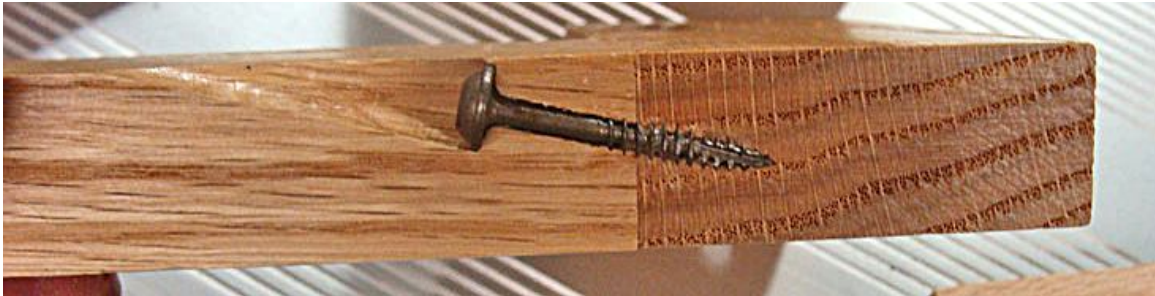
Typical pocket screw installation
